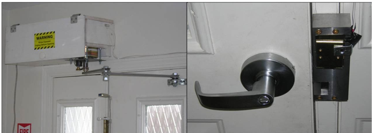
Fig. 9.2. Box Containing the Motor and Clutch (Left) and Replacement Strike Plate with Sliding Latch Mechanism (Right).
